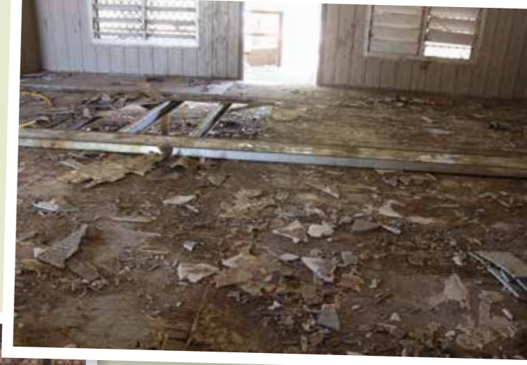
The house before the Fair Tradies helped us with renovations.
