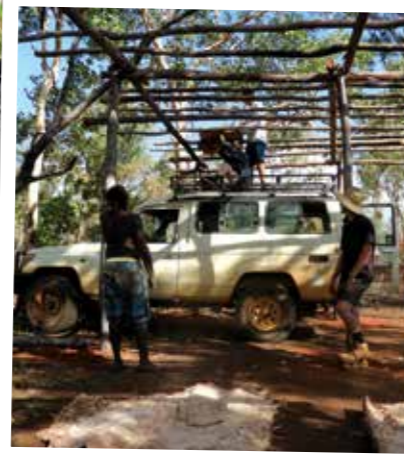
The yawurrinj hard at work building a new kunkodbarre.
